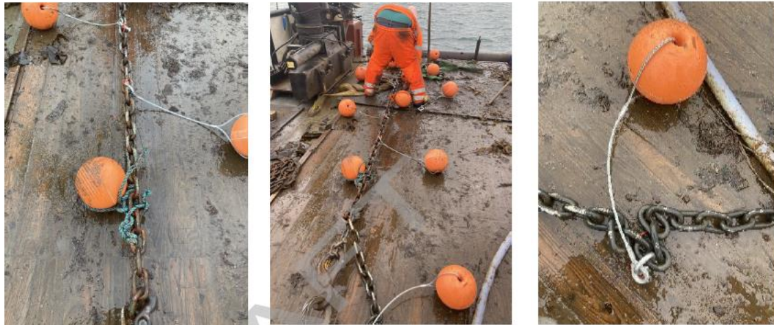
Photo: Rope ties, and then replacement galvanise wire on Stirling type moorings in Strangford Lough (Dr Rachel Millar & Dr David Smyth (on behalf of Cuan Marine Services))
