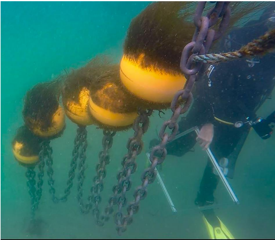
Photo: Stirling AMS in Cawsand (Plymouth) showing the mid-water floats attached to the riser (Mark Parry, Ocean Conservation Trust).
