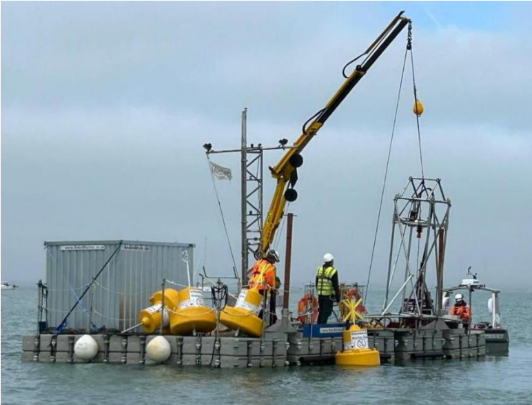
Photo: Mooring installation tool (ABC Subsea consortium)
